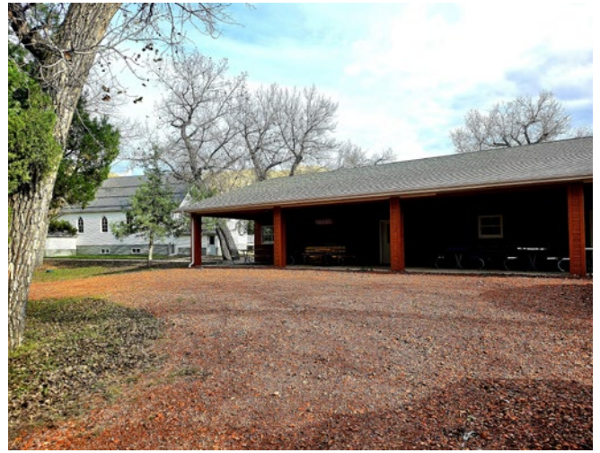
▲ Scoria loop created in front of staff/canteen building.
