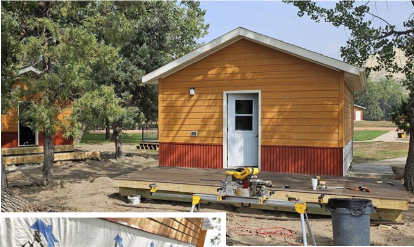
▲ Camper cabin getting a concrete foundation and a new deck.
