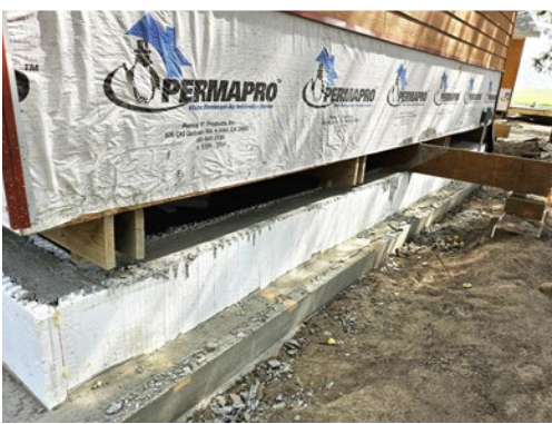
▲ Camper cabin getting a concrete foundation and a new deck.
